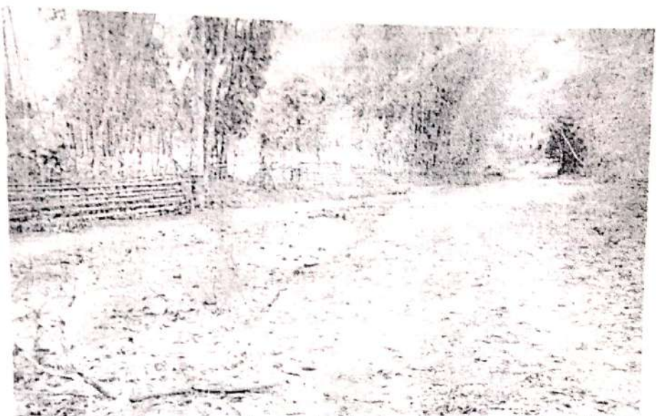
Picture:7: The raised level of the river bed due to mixing RBM with of muck/debris dumped by Shivam Trans Construction Private Limited. The raised level of river bed has changed the course of the river, letting them into the paddy fields of the local poor people.
